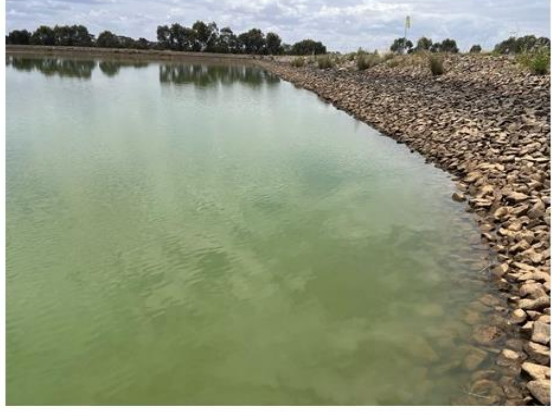
In drinking water reservoir
